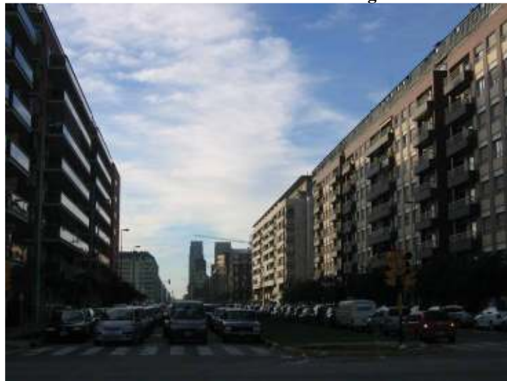
Picture 4: New construction in Puerto Madero along the Southern Coastline
